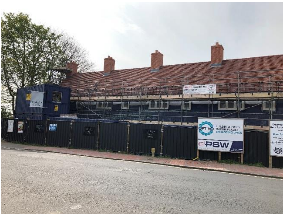
Cottages – battening for tile hanging started
