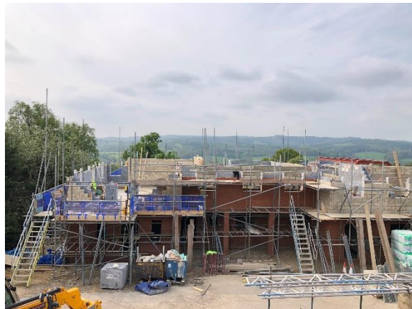
Flats – brickwork continuing
